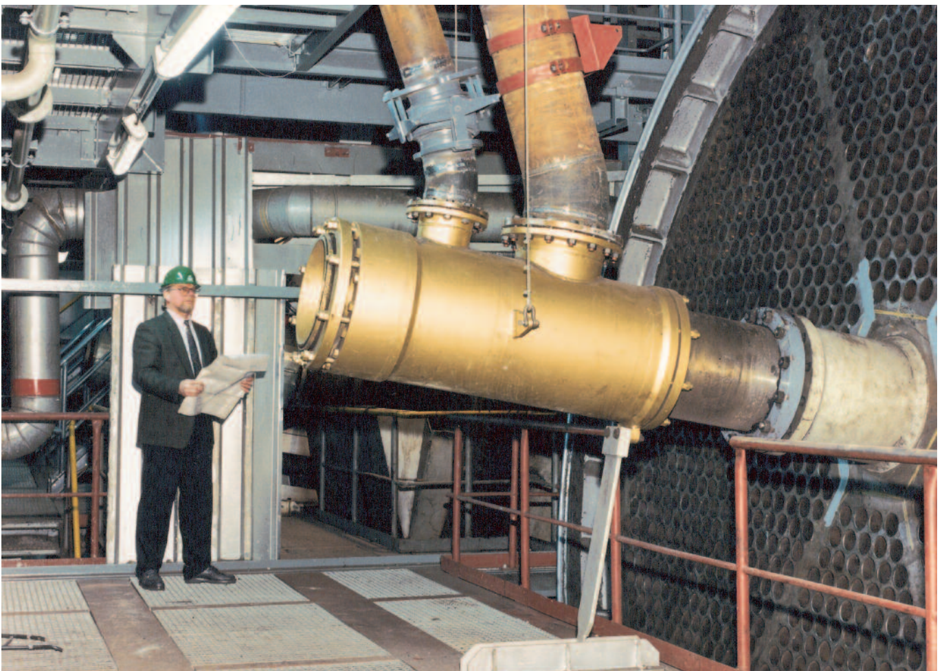
Series H + DC: Especially suited for large steam capacities; available diameters up to DN 350.
